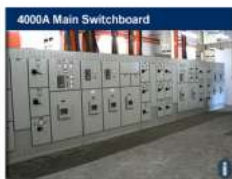
4000A Main Switchboard
