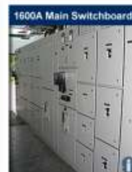
1600A 2 Incomer Main Switchboard
